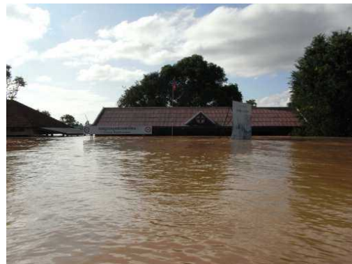
Flooding due to water release from a dam (Cambodia)
