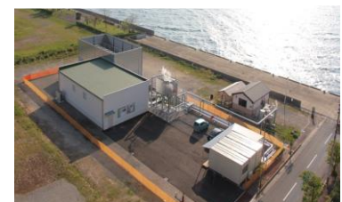
A complete view of the Obama-Onsen Binary-Cycle Power Station.
